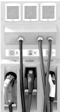
Figure 7 Charging options for electric vehicles and "vehicle connection to a Combo 2 fast charging station"
